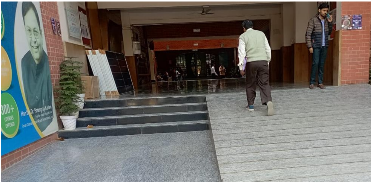
Photo: Screenshot of Ramp Facility
