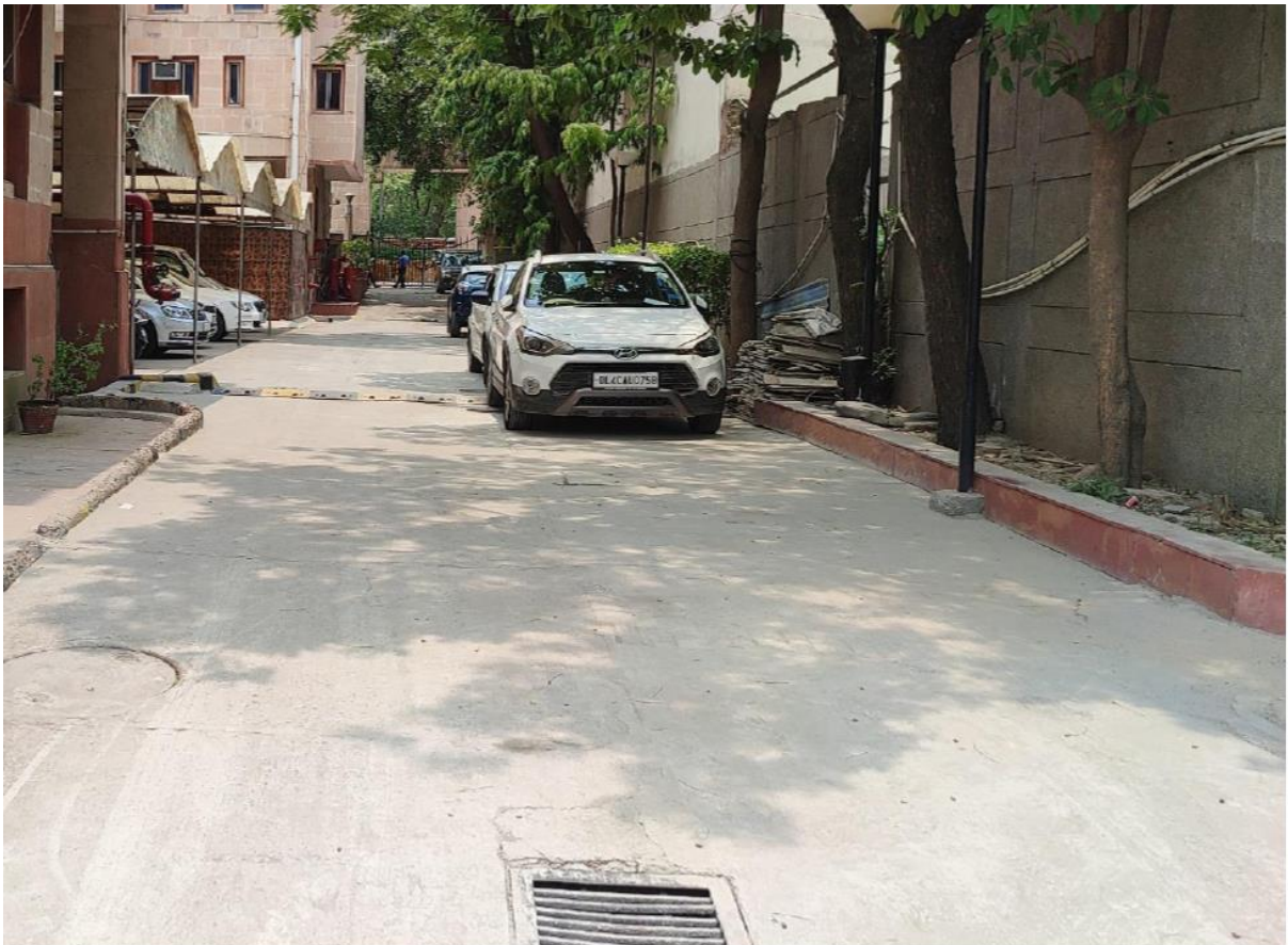
Photo: View of All Weather Approach (Road)
